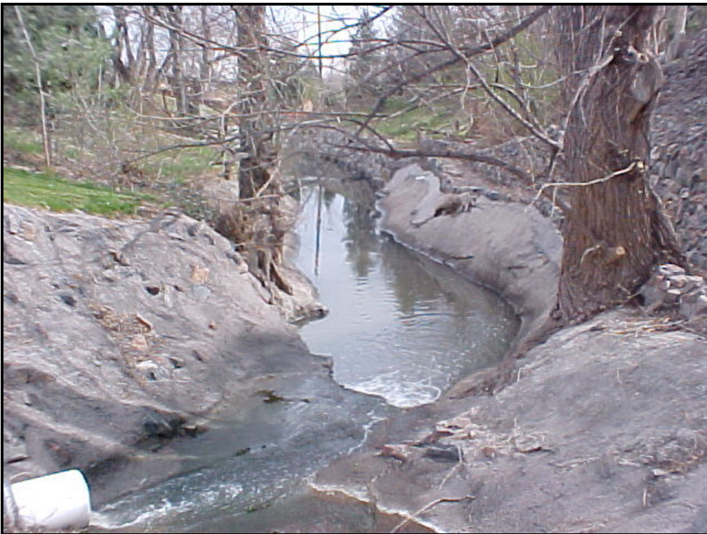
Figure 8 – Looking Downstream from Pond Outlet
