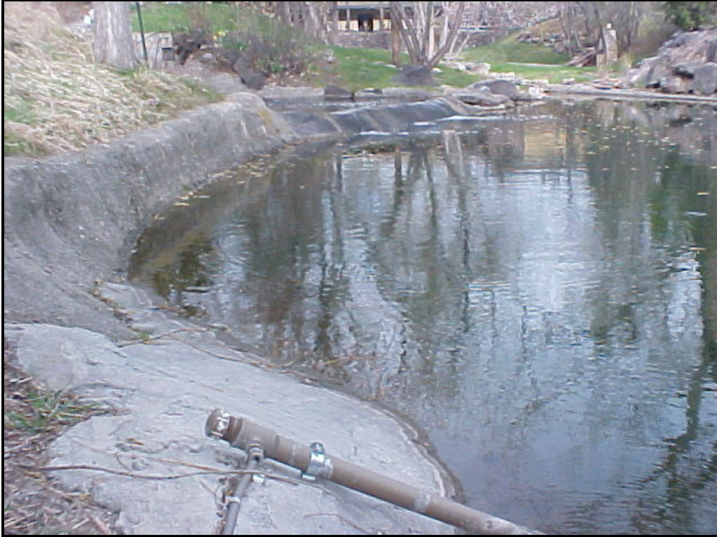
Figure 7 – Looking Upstream at PT Tube
