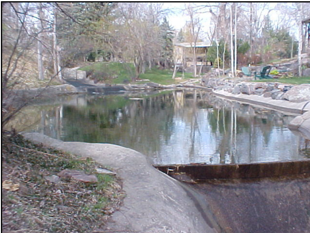
Figure 6 – Looking Upstream at Pond Inlet
