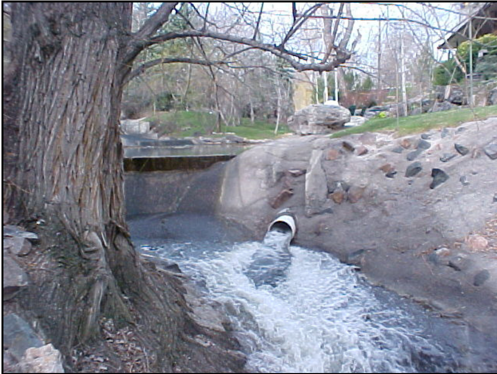
Figure 5 – Looking Upstream at Pond Outlet
