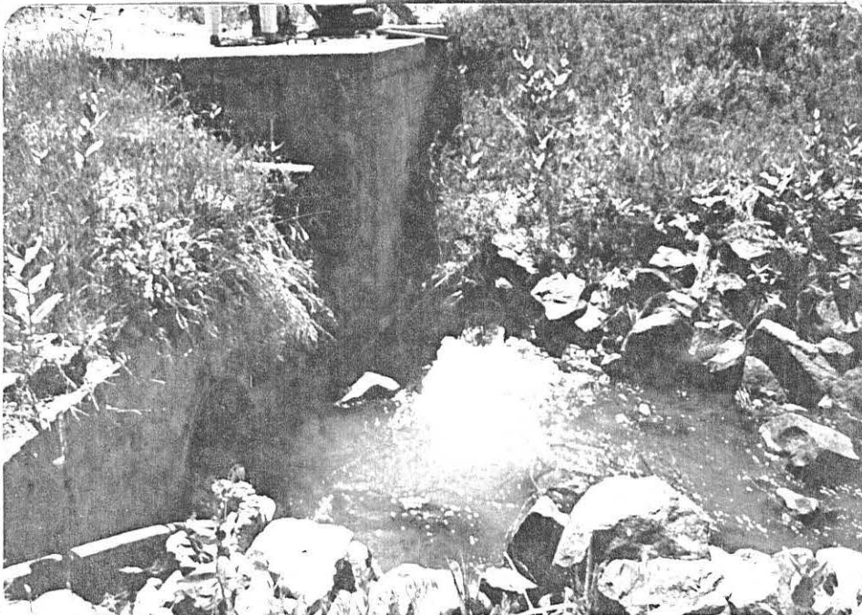
Photo No. 11 Irrigation ditch outlet and stilling basin adjacent to gate house.
