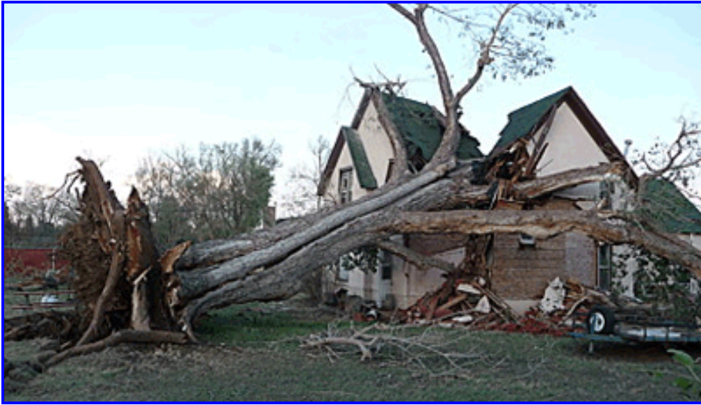
Figure 5: Damage caused by straight-line winds on July 20, 2009 in Wheat Ridge, Colorado
