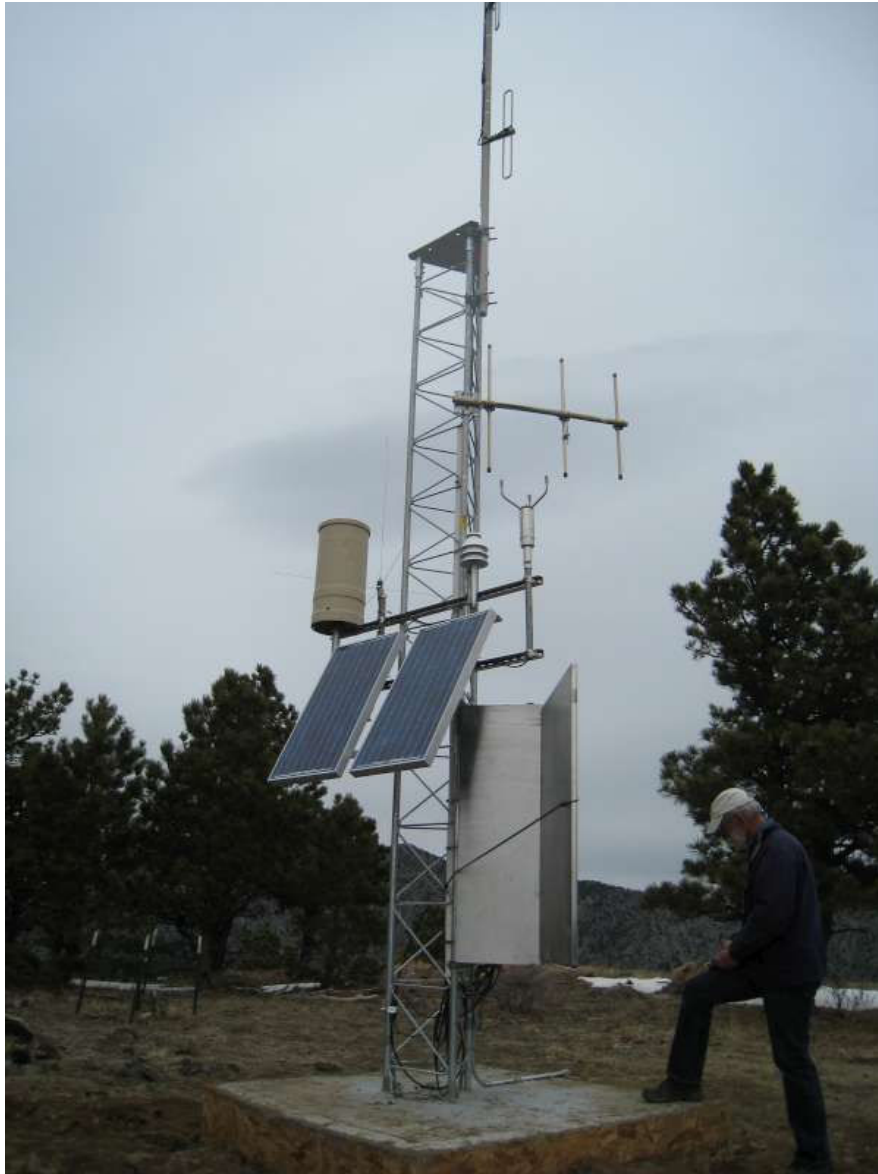
Figure 10: Current Blue Mountain Installation
