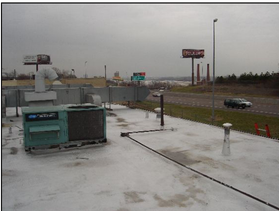
1 ≡ Gage site problems, any information would be completely unreliable (gage located on top of AC unit)
