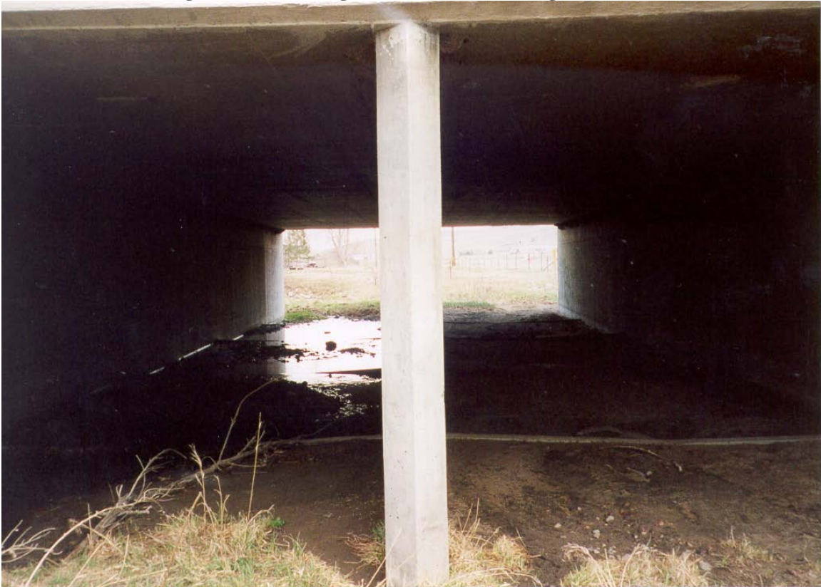
Figure – 5 Looking Downstream Through Culverts
