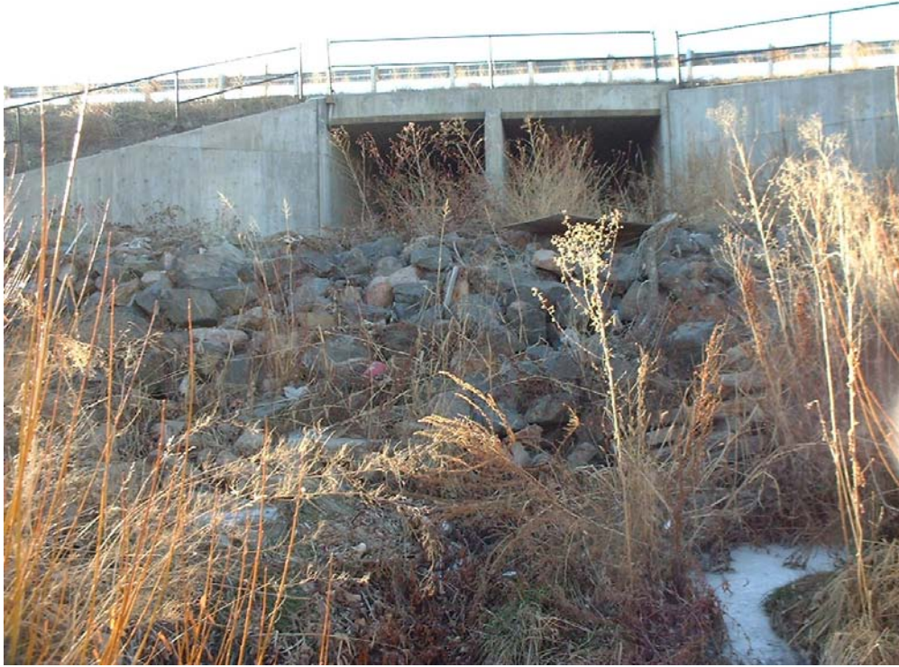
Figure – 5 Looking at Downstream Outlet of Culverts
