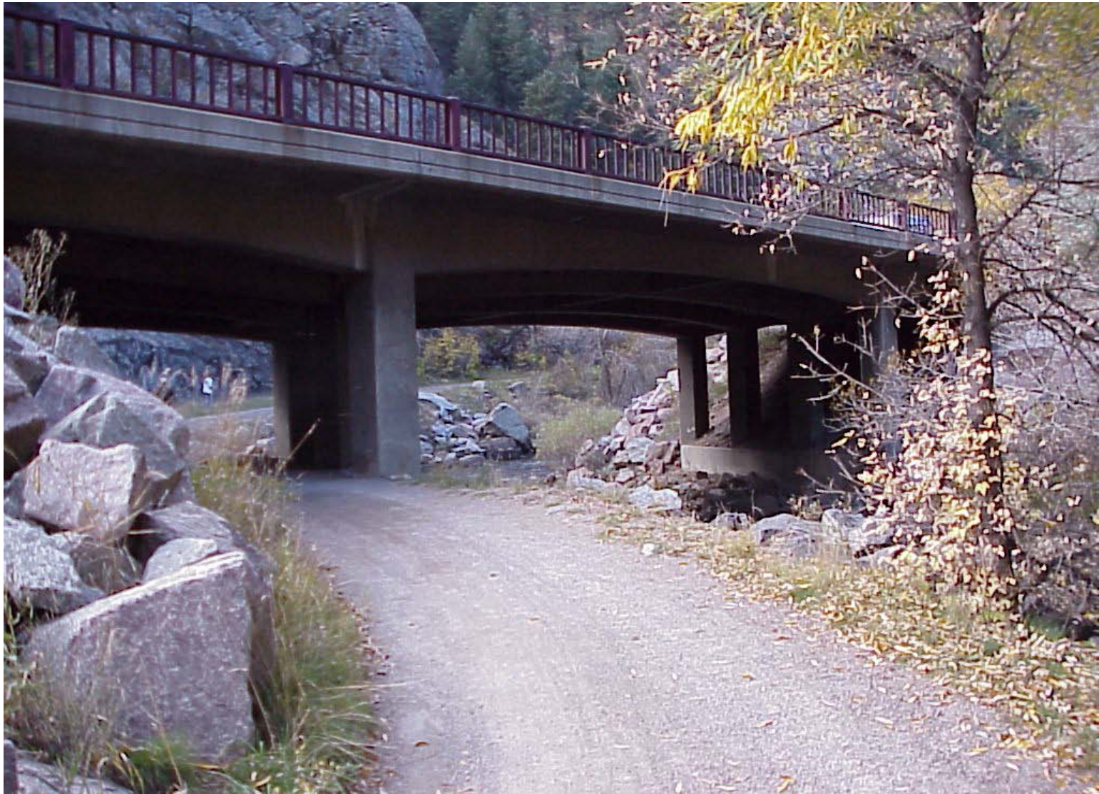
Figure – 5 Downstream face of bridge
