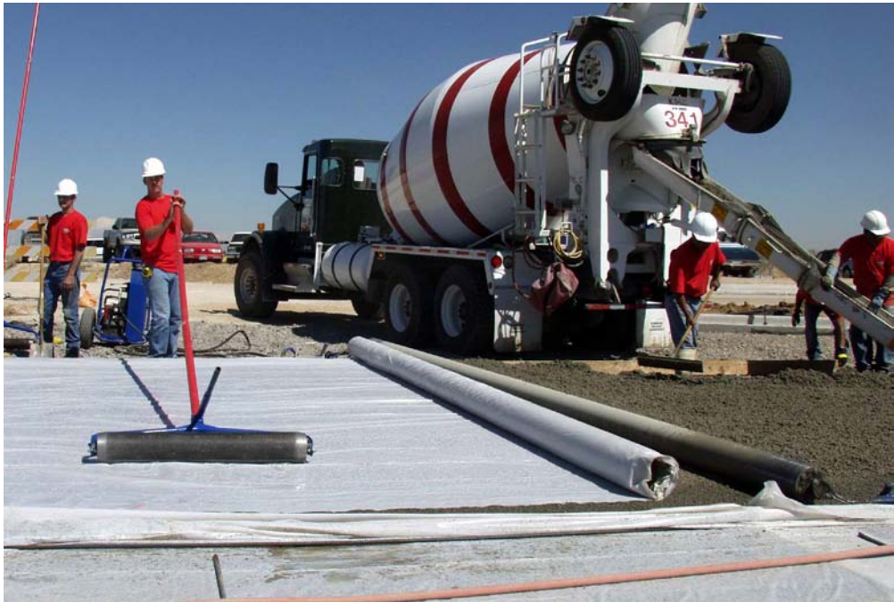
Figure 2. Cross Rolling Pervious Concrete
