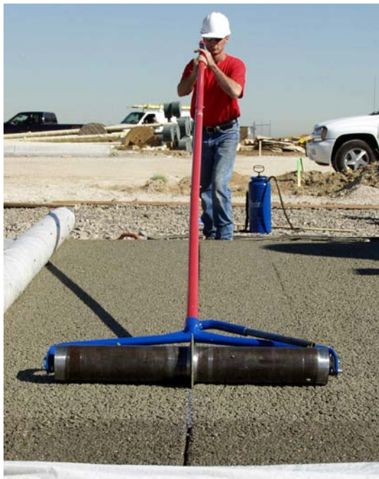
Figure 3. Pervious Concrete Jointing
