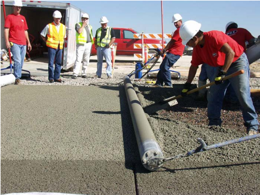
Figure 1. Roller Screeding Fresh Pervious Concrete
