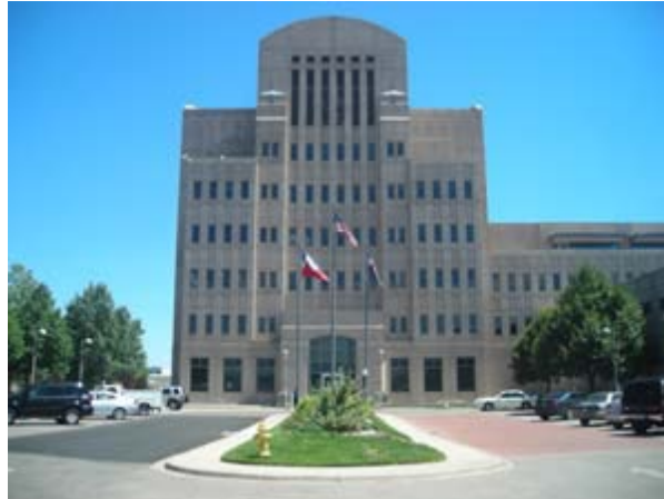
Photograph 2. Denver Public Works Building (Left of island: porous asphalt, right of island: PICP).
