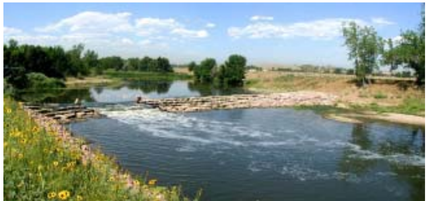
Before and after views of the gage control section
