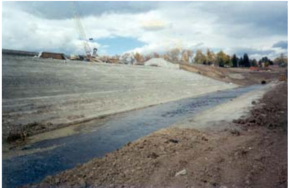
The Leyden Lake project features a 380 feet wide roller compacted concrete spillway with a capacity of 75% of the probable maximum flood.
