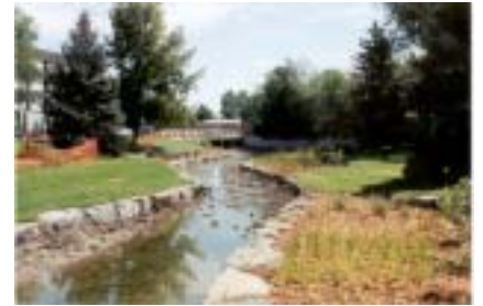
Immediately after construction
