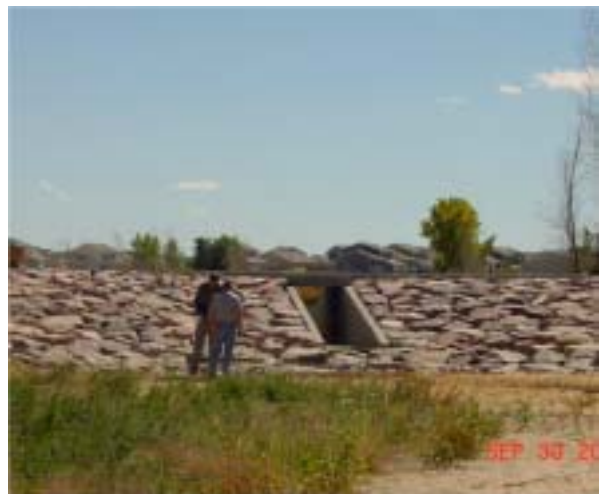
Parkfield Lake spillway.
