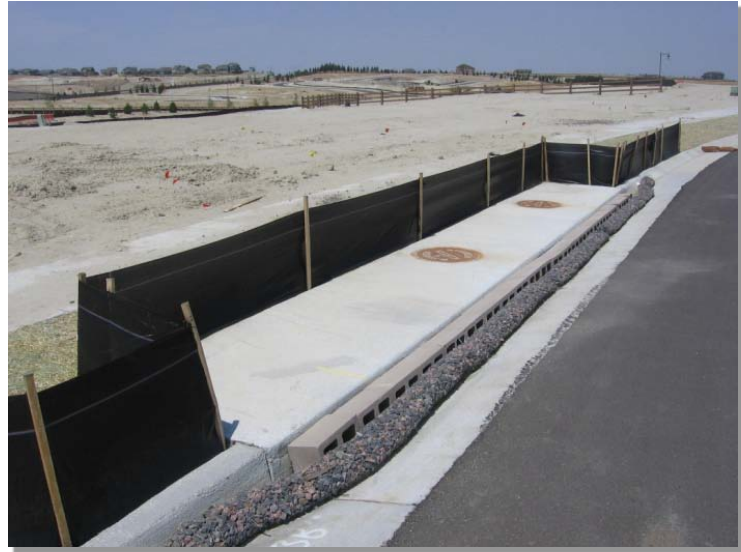
Photograph IP-1. Inlet protection for a curb opening inlet.
