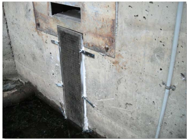
Photograph OS-3. Trash rack after repair.
