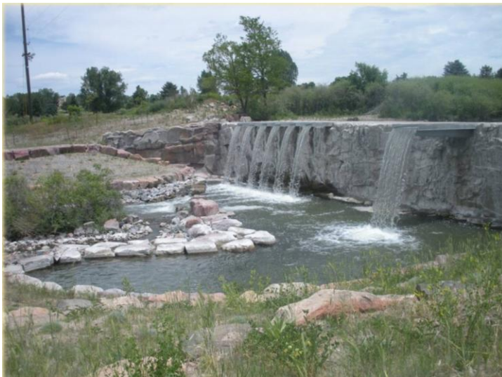
Cherry Creek Drop Structure No. 27 in Denver
