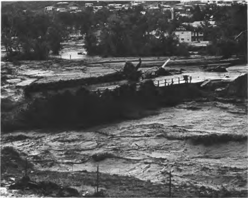
FIGURE 9.—Bridge on approach road from Castle Rock to Interstate Highway 25 destroyed by East Plum Creek. Denver Post photograph by William Peters.
