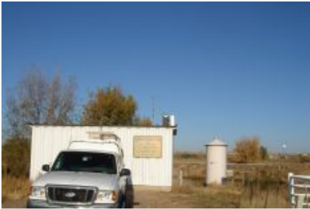
1660 - SPR at Henderson - a
