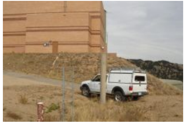
4100 - Filter Plant - b
