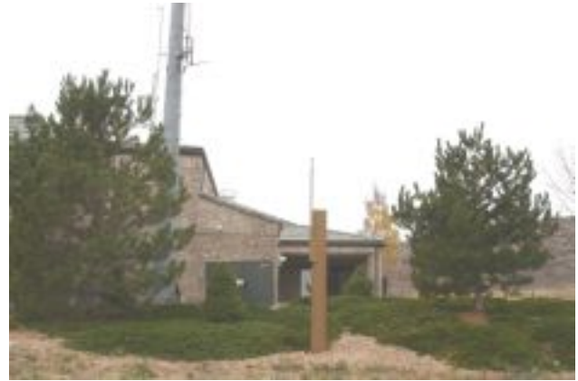
1370 - Fire Station 13 - b
