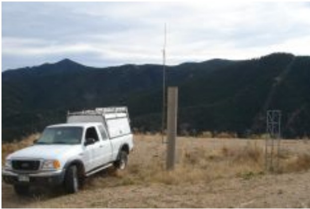
4100 - Filter Plant - a
