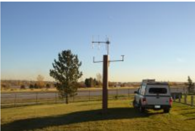
2710 - Highlands Ranch WTP - c
