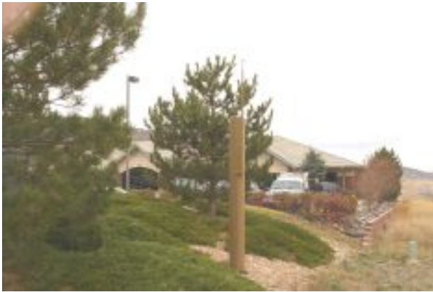
1370 - Fire Station 13 - a
