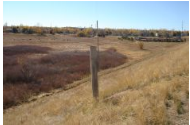
1600 - Englewood Dam - b
