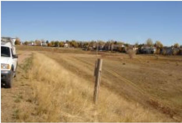
1600 - Englewood Dam - a
