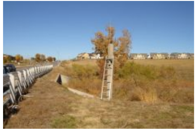
820 - ETG @ Buckley - b
