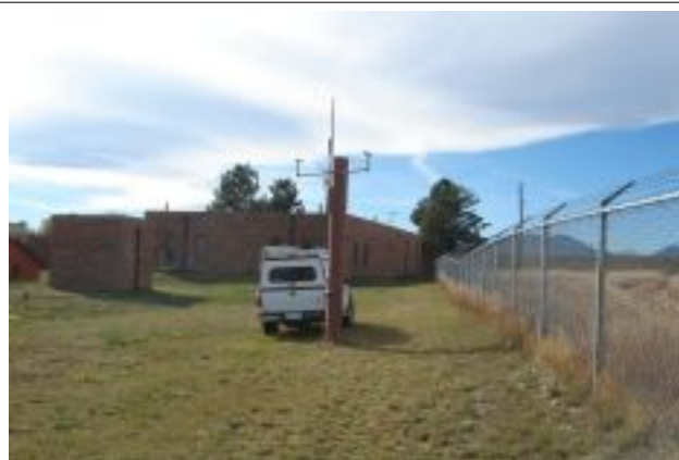
4750 - Louisville WTP - b
