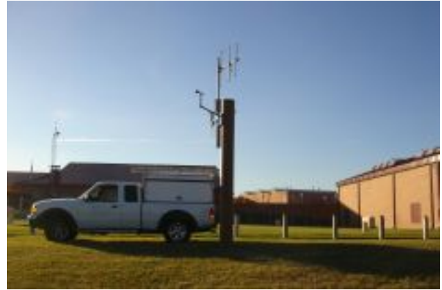
2710 - Highlands Ranch WTP - b
