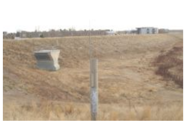
410 - Kelly Dam - b
