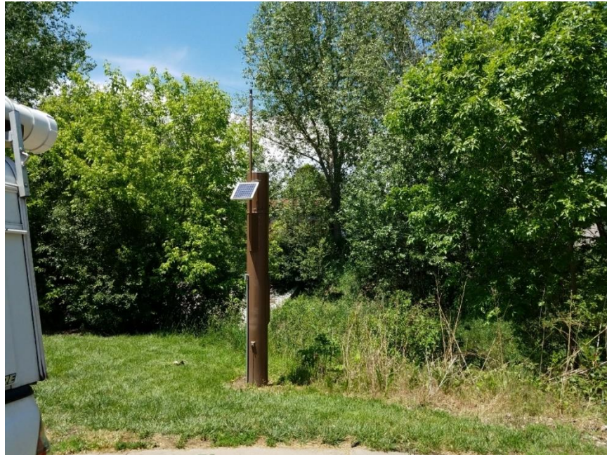
Figure 3-2: Weir Gulch Station
