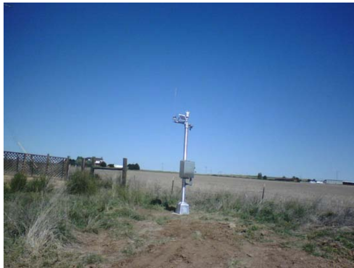
Figure 6: Pump Station #3 (Aurora Airpark)
